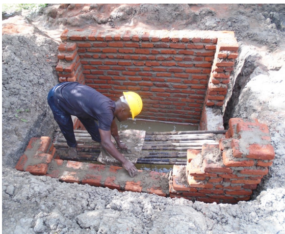
Left: Building up the pit lining.
