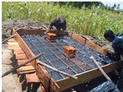
Below—preparing the concrete slab.....
